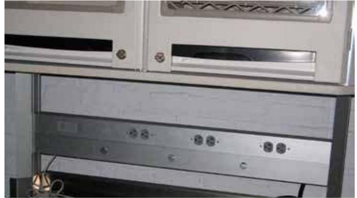
Double Raceway attached to a mobile Starsys system.
